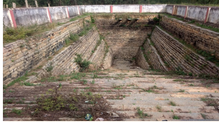
Old structure (Kalyani) at Jadigenahalli Gram Panchayat
