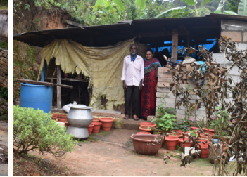
House damages due to landslide in Kodagu
