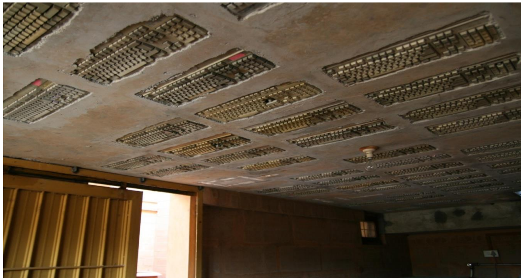
Photo 1: Using Disposed of Keyboards to Design Creative Roofs, Bangalore, S Vishwanath
